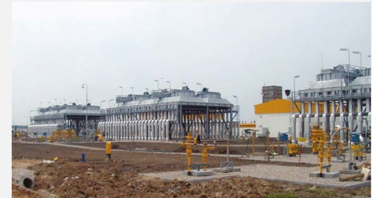
Figure 1. Construction of a new natural gas storage facility.
