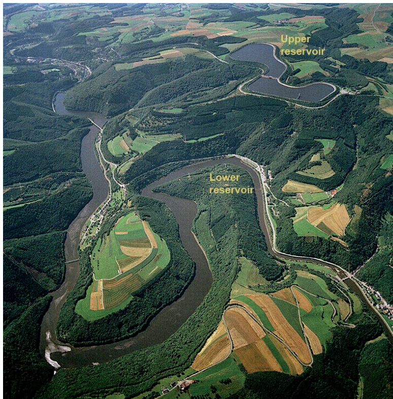
Fig. 1: Aerial photo of the separate upper and lower reservoirs along with the dammed course of the river (Our) in Vianden (Luxembourg).
